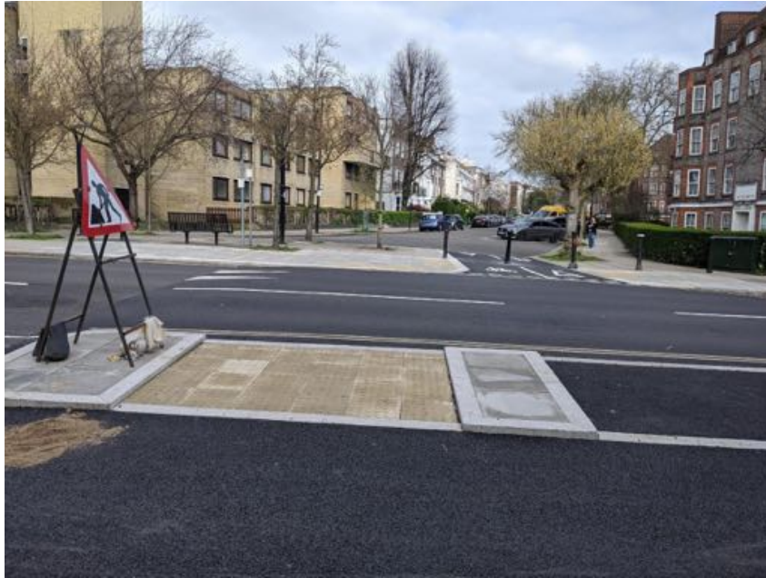
View to Queen's Crescent from WB track
