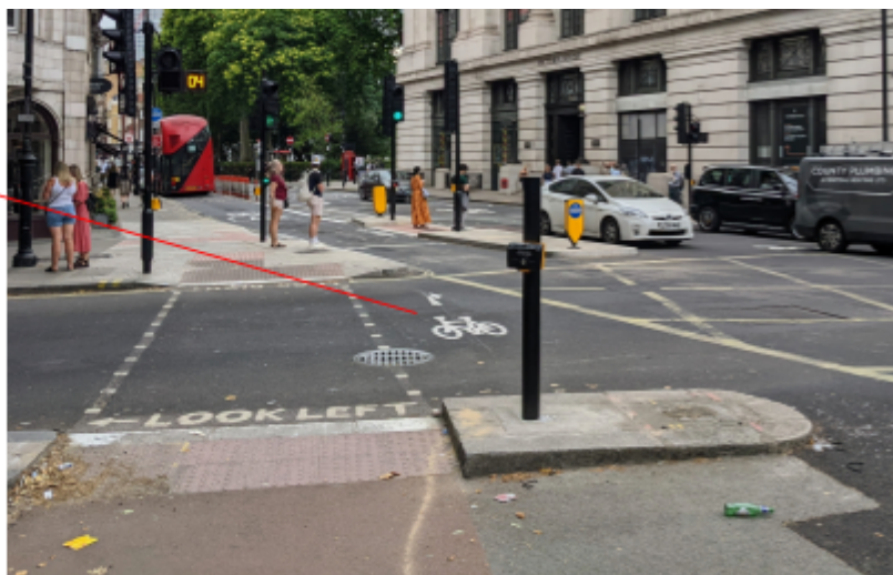
Photo 2: Two-stage right turn area in front of Southampton Row (N) with Theobalds Road ahead. Needed because Vernon Place has an early release. See Section 2.4
