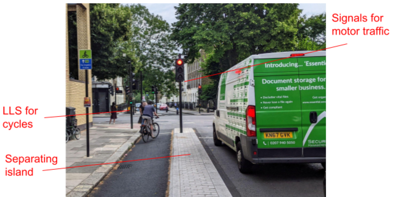
Photo 5. Sidmouth Street approach to GIR – a dedicated signal stage.
