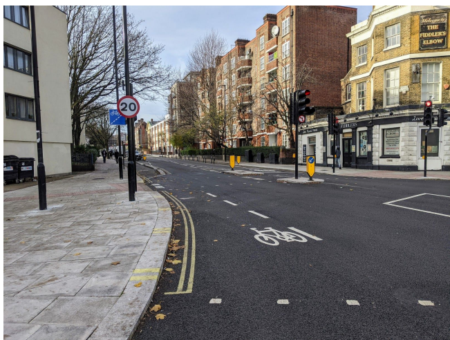
Figure 11. Western exit from Malden Road junction: advisory marking up to the pedestrian crossing and kerb protection immediately after
