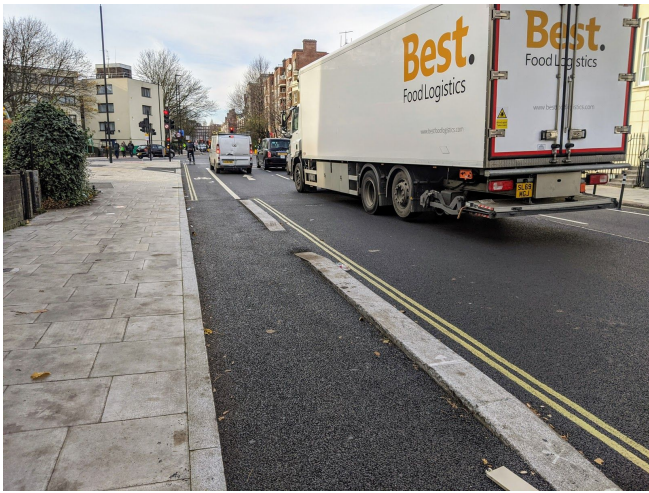
Figure 7. Westbound approach to Malden Road. The concrete kerbs stop short of the junction; after that the marked lane is unprotected and narrows down to about 1.5m.
