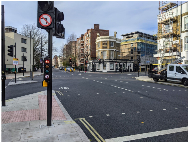
Figure 10. Close up of Malden Road junction showing the low-level lights and the two-stage right turn
