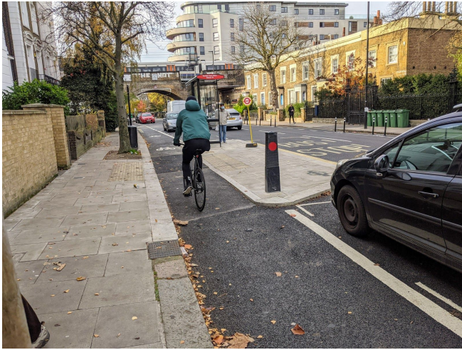
Figure 3. Bus stop near Hadley Street. Needs zebra and other markings.
