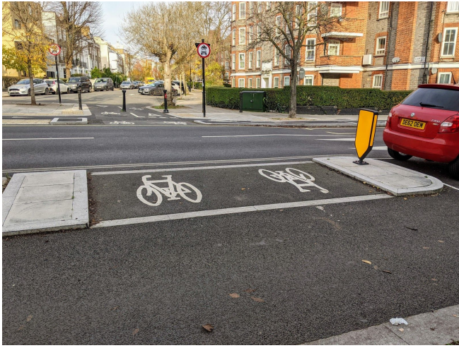
Figure 12. Queen's Crescent Junction. Waiting space for cyclists entering and leaving the cycle lane on both sides of the road
