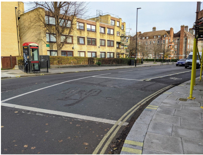
Figure 14. Haverstock Hill junction. Stepped track reaches ASL box. ASL box needs logos
