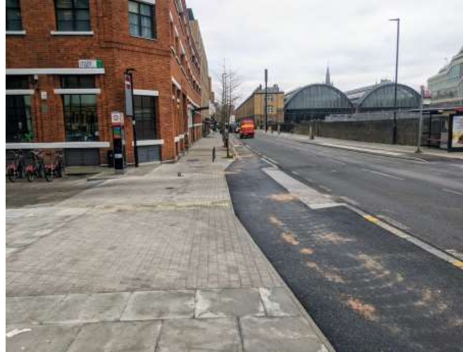
Blended junction at Crinan Street
