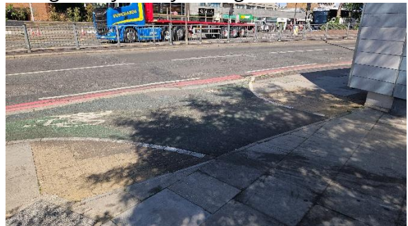
Fig 2.4: paving change of cycleway
