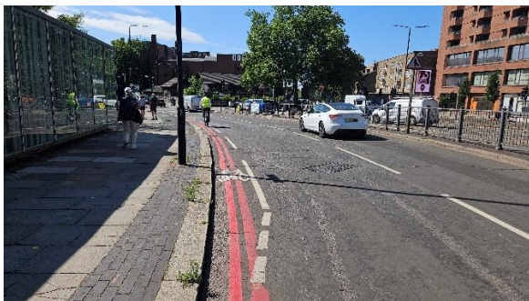
Fig 2.8: v. narrow feeder lane to exit at 2
