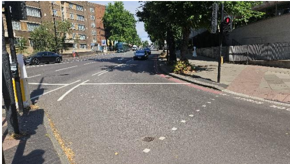
Fig 16.3: north from Adelaide Road (e, 16)
