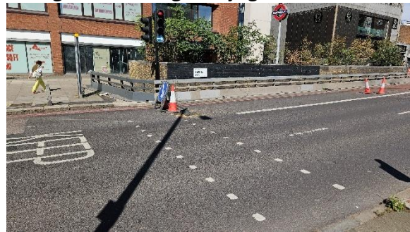
Fig 3.4: carriageway join from refuge 2
